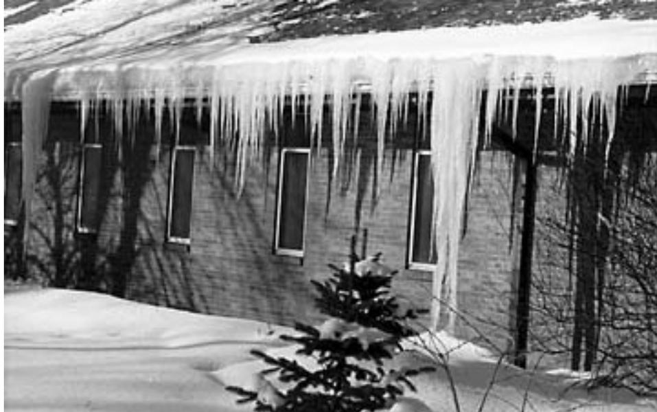
During the blizzard of 1994 in Maryland, thousands of homes and commercial properties dealt with damages from heavy accumulations of snow, which caused a large number of roofs to collapse from the weight of the snow. At the beginning the concern was the amount of weight on the roofs, but that quickly shifted to ice dams as the snow started to melt and refreeze.
