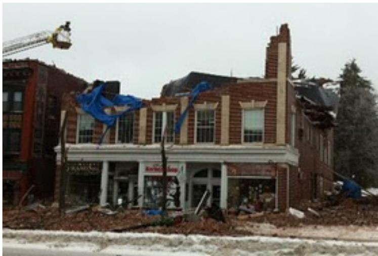
washer like this is a recipe for disaster! If you spray water on the roof it will usually refreeze immediately, which will only add more weight to the roofing support structure that may already be over capacity.
